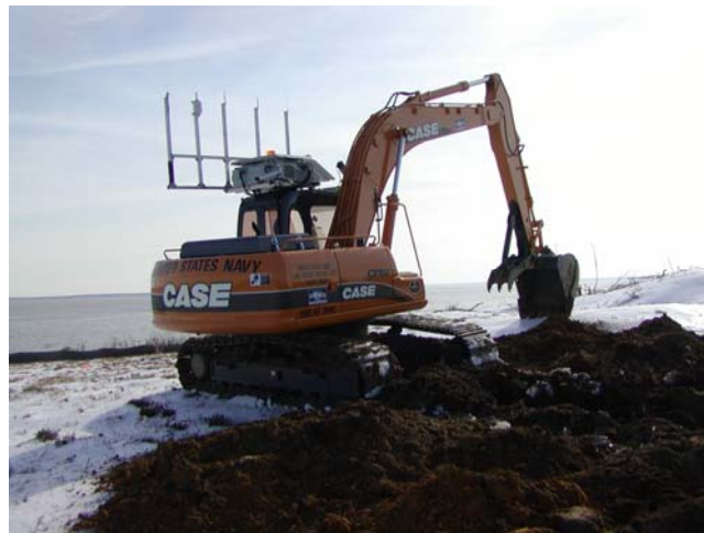
Fig 2. Remote-Controlled Case Excavator
